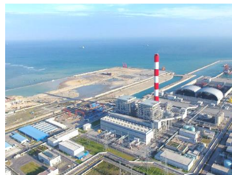
Vinh Tan 1 coal-fired BOT power plant, Vietnam. 2x620MW, COD 2018
