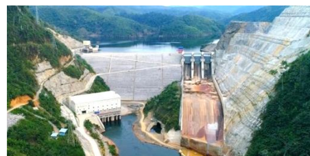
Nam Tha 1 hydropower BOT project, Laos. 168MW, COD 2019
